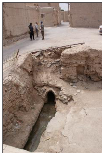
Mansouran Ditch, one of the Branches of the Mohammadiyah Na'een qanat.
